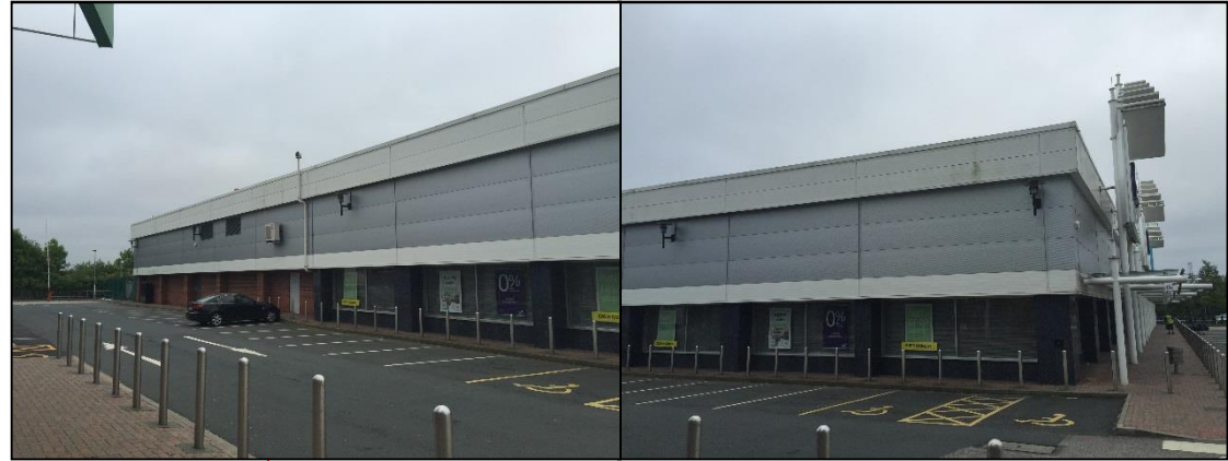
Side Elevation (North): no signage
