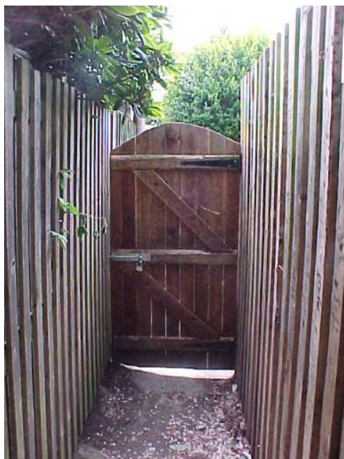
Forbidding, enclosed appearance, typical of communal rear access footpaths
