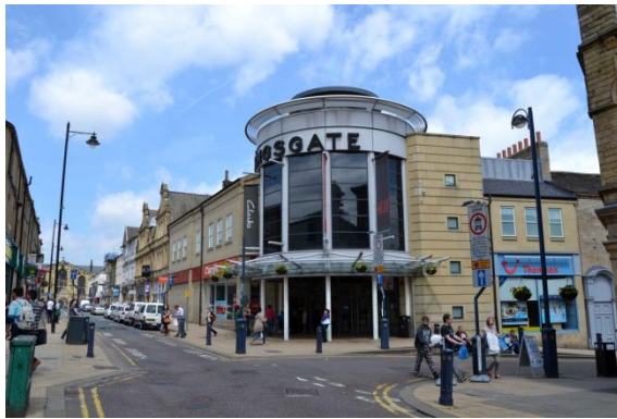
Photo 3 – Existing Kingsgate Centre Entrance
