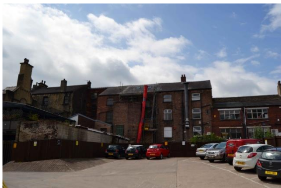
Photo 5 – Rear of 20 - 22 Cross Church Street
