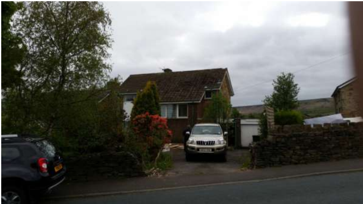
View of existing front house(plot 1) with existing vehicular access
