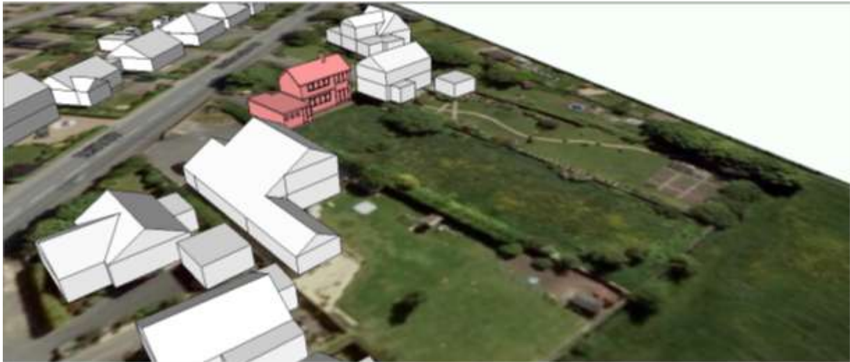
Aerial view of the existing front house
