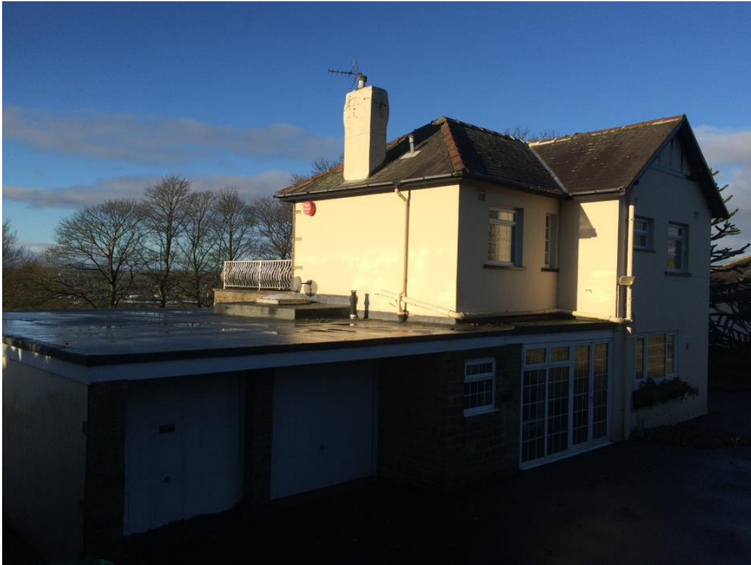
Photo 5. Rear elevation of house viewed from east
