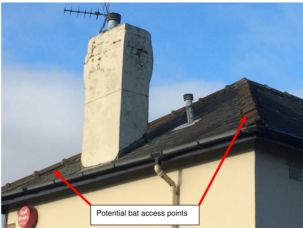
Photo 6. South-east facing hipped-gable viewed from east
