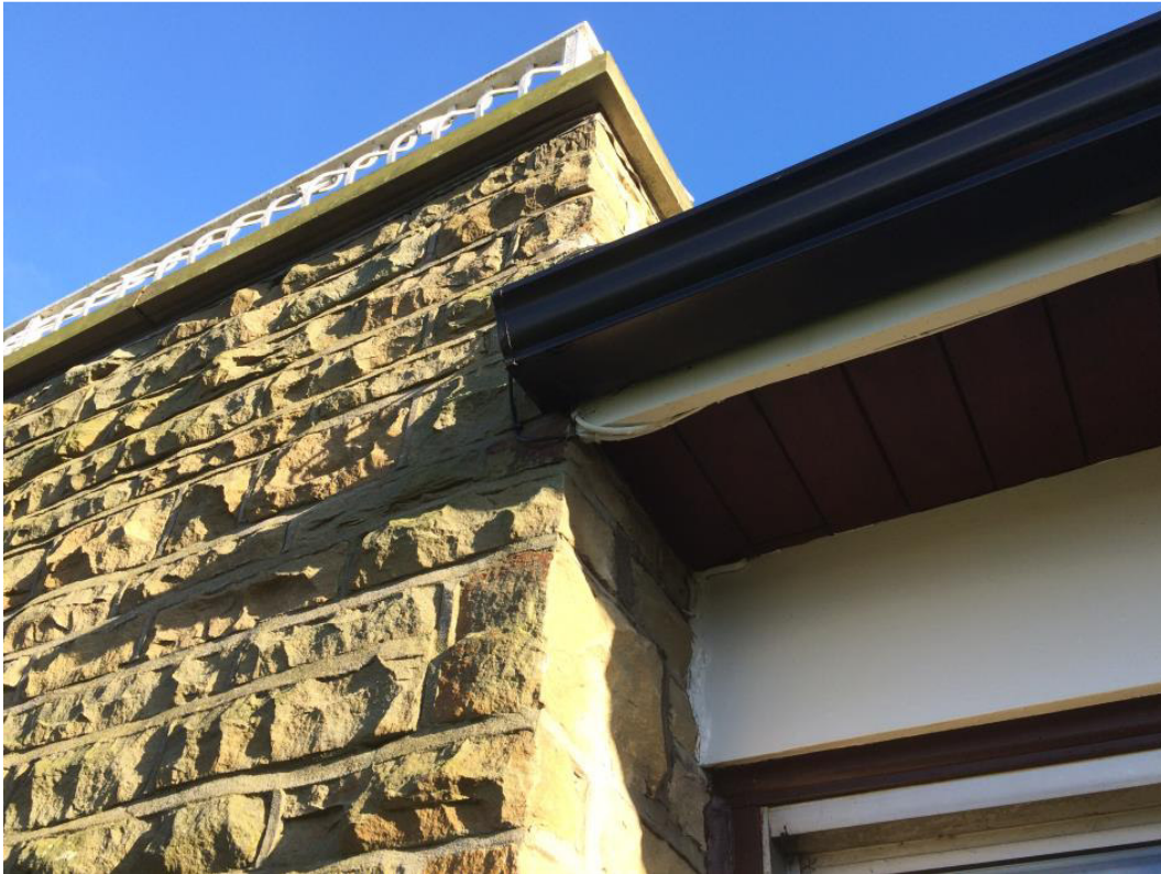
Photo 3. Detail on south-west elevation showing flush soffits and roof verges
