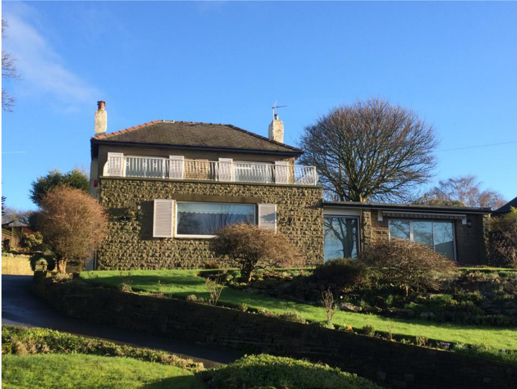
Photo 1. 333 Drub Lane viewed from south-west (front)
