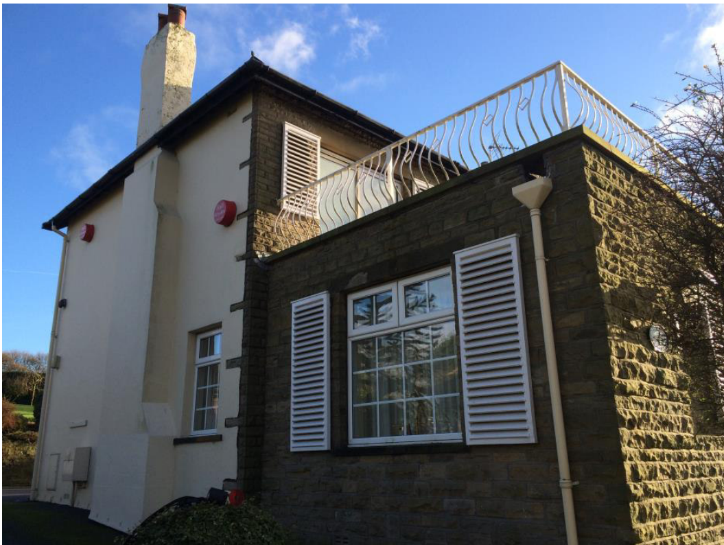
Photo 2. North-west elevation of house viewed from west
