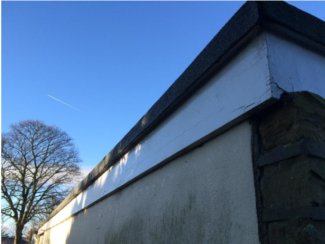
Photo 7. South-east elevation of house showing eaves boards in good condition and flush with wall providing no potential bat access points
