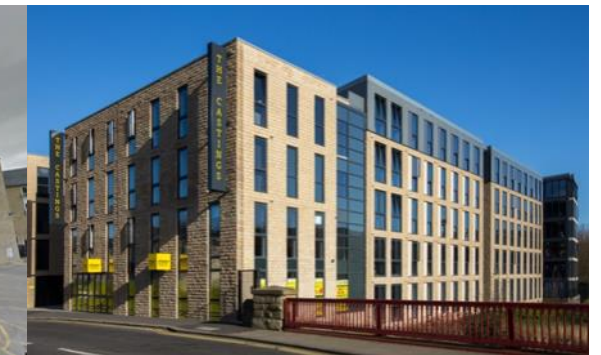
Fig 7: The Castings Student Accommodation
