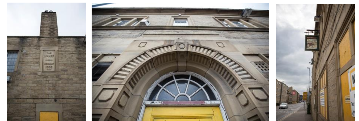
Fig 12: Existing architectural features of the Public House
