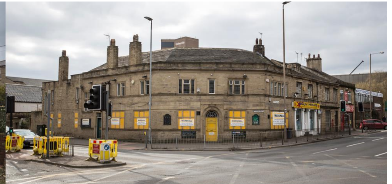
Corner of Wakefield Road and Firth Street
