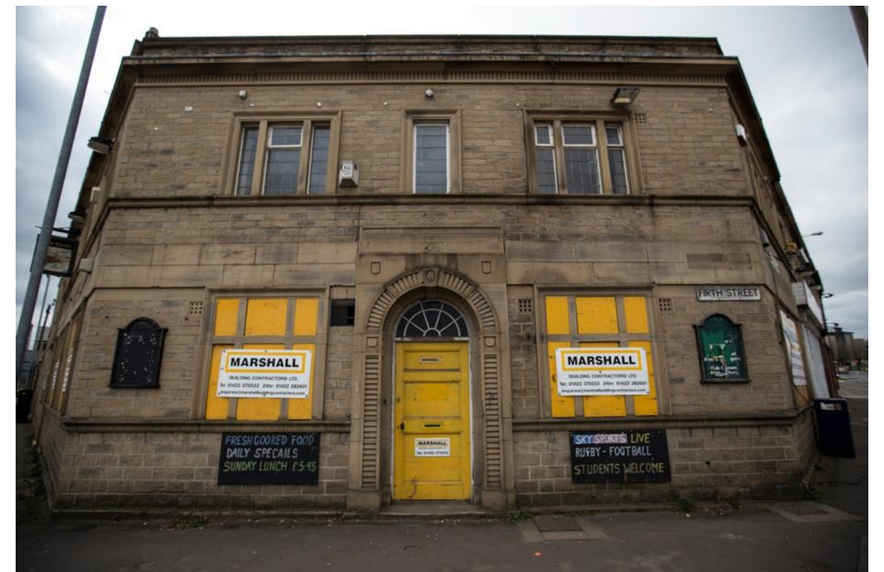
Fig 11: Existing Stone Facade of the Public House
