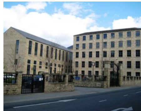
Fig 5: Aspley House Student Accommodation
