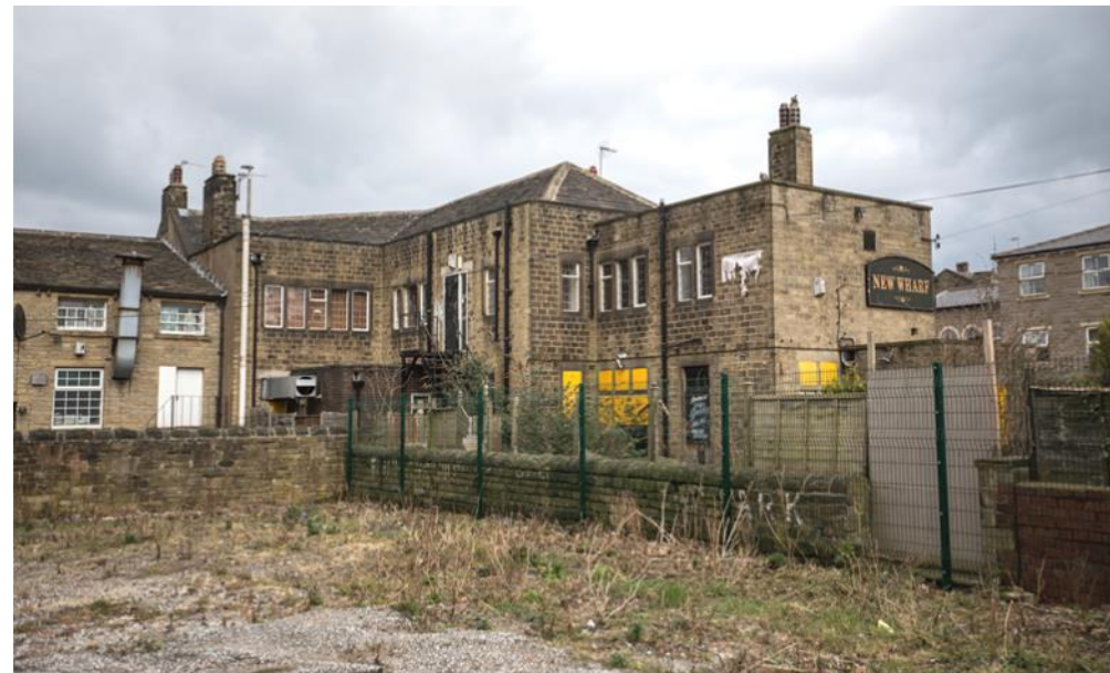
Rear of Site from Sand Street
