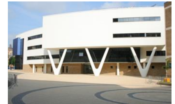
Fig 4: University of Huddersfield Creative Arts Building
