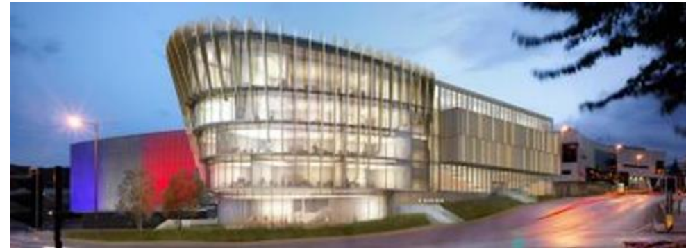
Fig 3: University of Huddersfield Shorehead Building (under construction)
