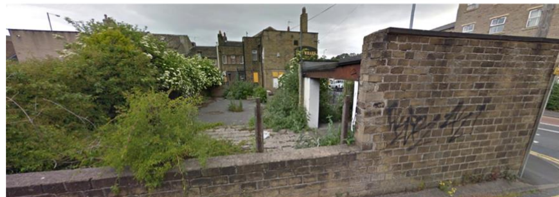
Rear boundary wall to Sand Street
