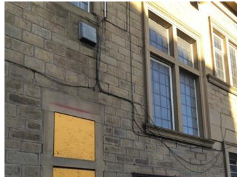
Fig 18: Existing fenestration detailing of Public House
