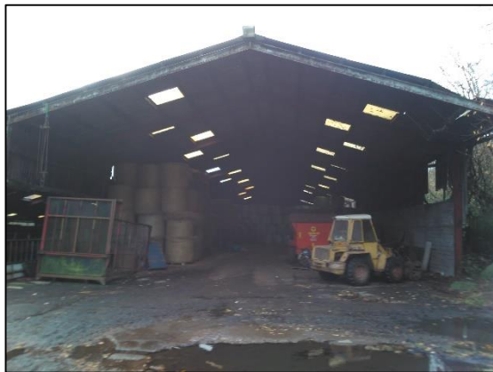
Photograph 18: Interior of Building 5
