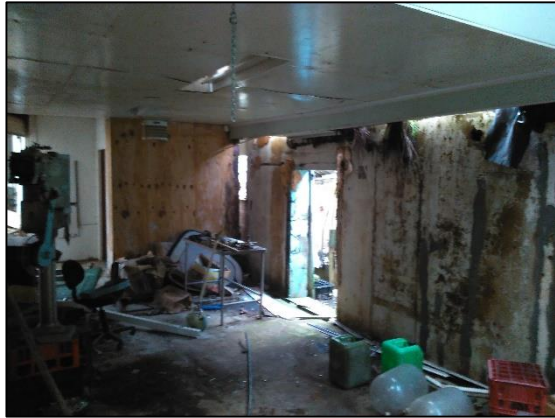
Photograph 16: Interior of Building 3, north
