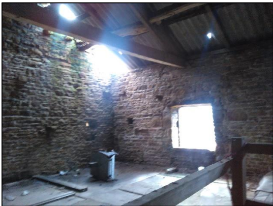
Photograph 11: Building 1, 1 st floor
