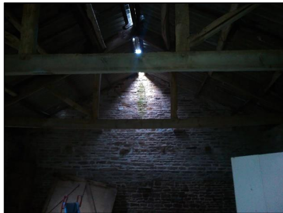
Photograph 12: Building 1, ridge board
