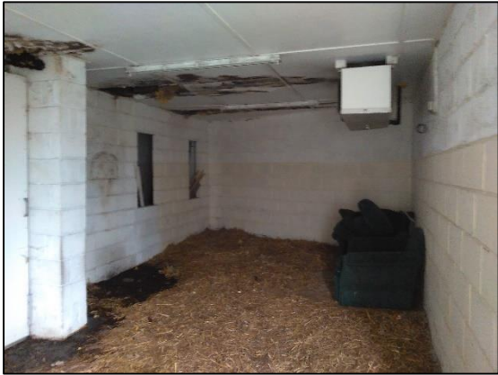
Photograph 15: Interior of Building 3, south
