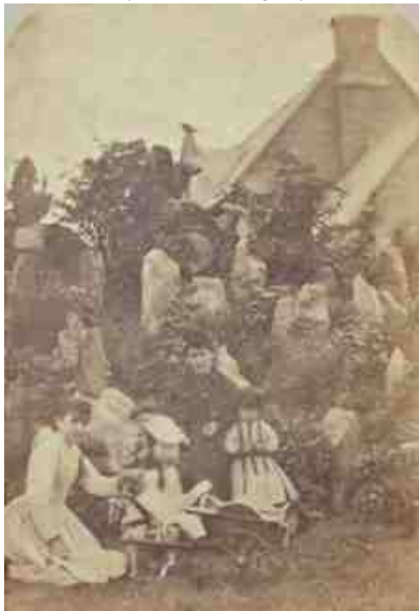
Fig. 7. Photograph dated 1867 with the stable block in the background.
