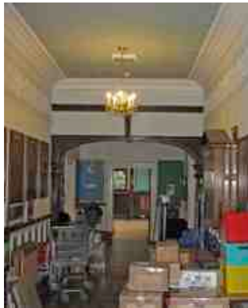
Fig. 31. Three centred arch between the original hallway and extension.
