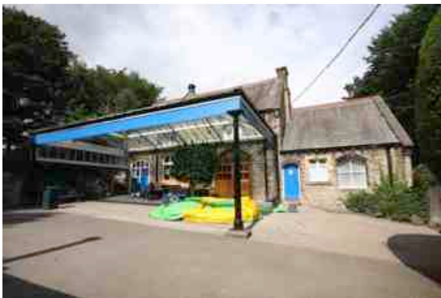
Fig. 73. Former stable block and canopy. The building is now used for classrooms
