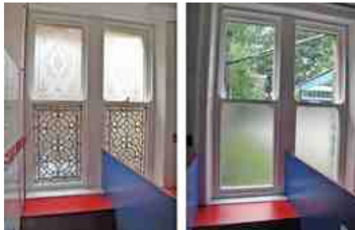
Fig. 50. Modern toilets in the 1903 addition. The sash window frames are original and the glass in the left hand window part of the historic fabric but the glass in the right hand window has Georgian wired glass.
