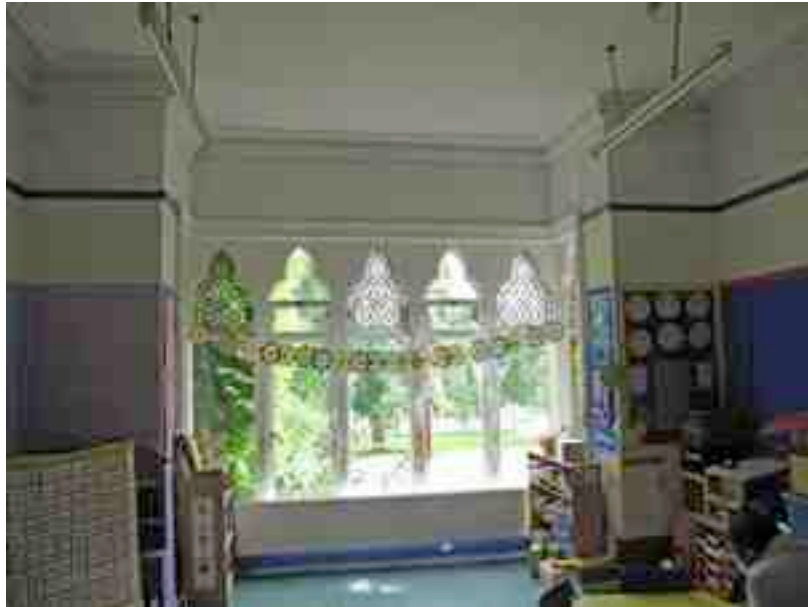
Fig. 35 Bay window to the classroom (003) which was probably the original dining room when the building was a house. Two of the windows have been adapted by the addition of casement lights.
