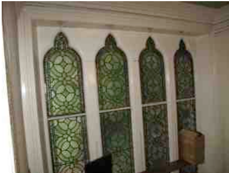
Fig. 65. Quarry glass windows with identical pattern found in the ground floor WC's (room 9 ground floor).
