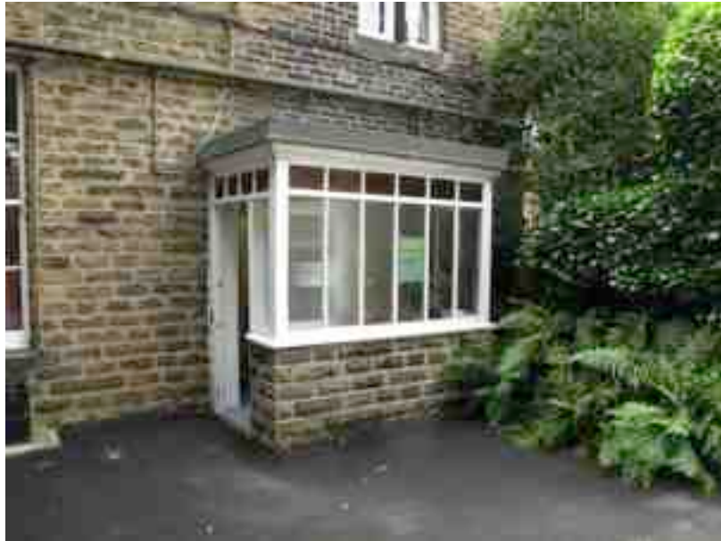
Fig. 21. Modern Porch to the the rear (servants/trade) entrance
