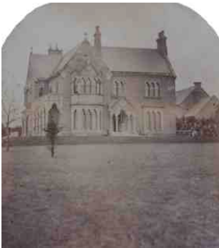
Fig. 2. Royds Mount taken 1867. Note stable block to the right of the picture. (Source: Mrs Hughes)
