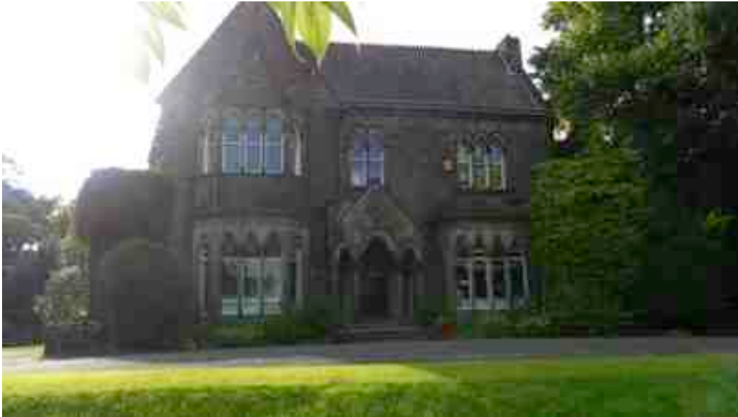
Fig. 17. The imposing main entrance - east elevation.
