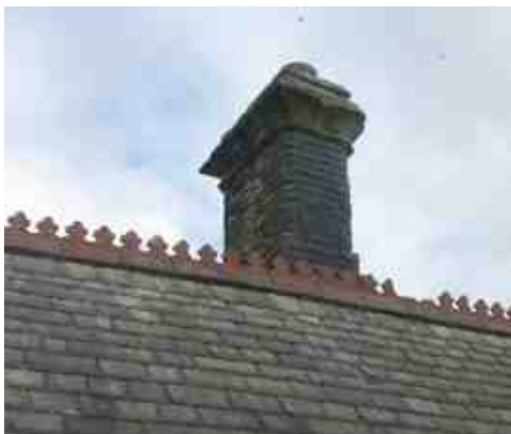
Fig. 16. Terracotta ridge tiles and chimney stack with a later pot.
