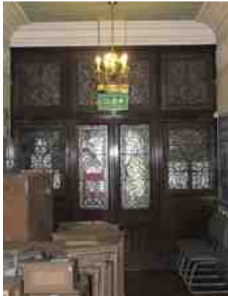
Fig. 29. View of the stained glass and timber frame separating the lobby and hallway. This panel may of been a later addition as the flow of the stained glass detail is more Art Nouveau than Gothic Revival.
