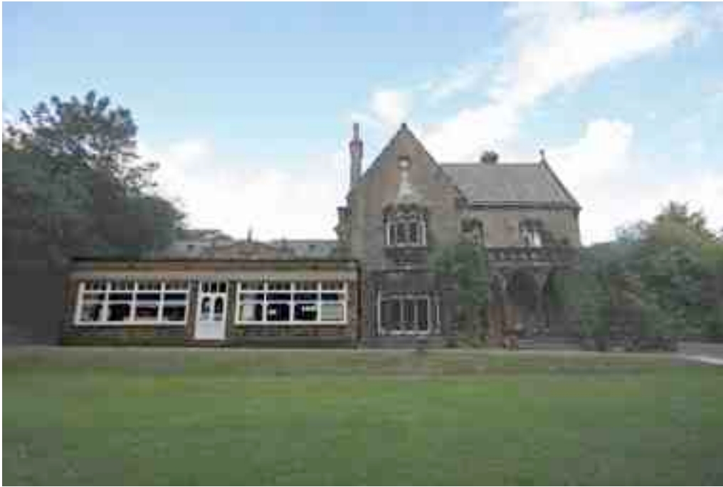
Fig. 19. 20th Century addition. Also note veranda and balcony to the main house.
