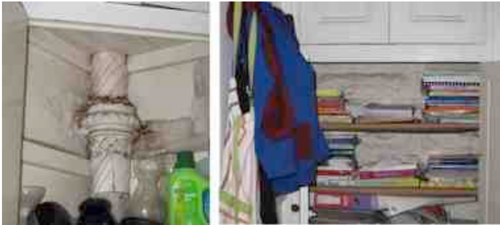
Fig. 46. Original fabric now hidden enclosed within two cupboards.
