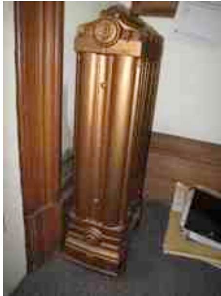
Fig. 64. Jobsons radiator located in the Bursar's office in the c.1893 addition to the north elevation.
