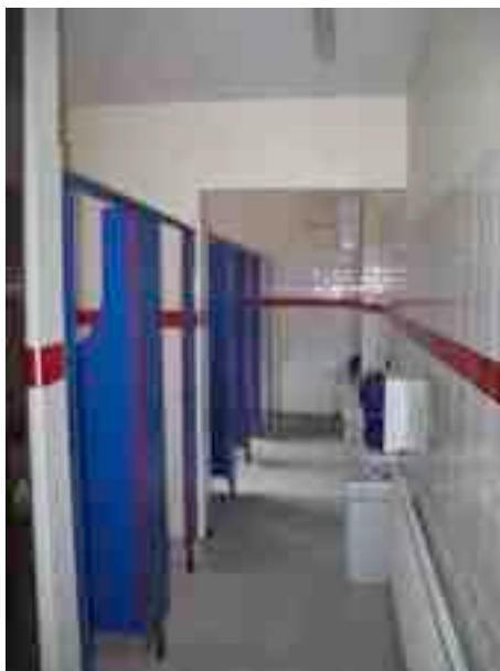
Fig. 51. Modern toilets in part of the Lunn's 1903 addition.
