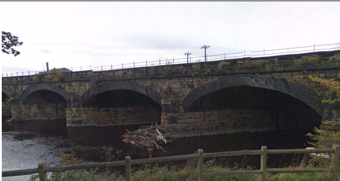
Figure 5.4: Railway Bridge approximately 940m east of development site
