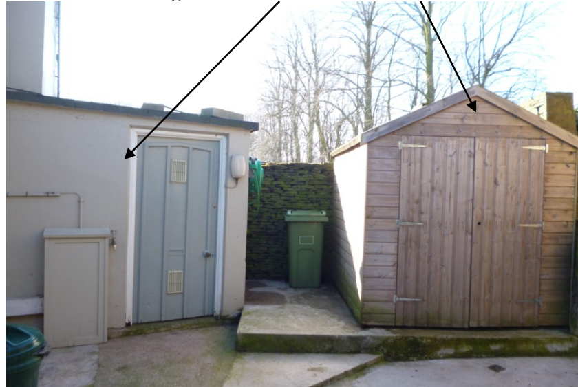
Figure 4 – Boiler house and shed
