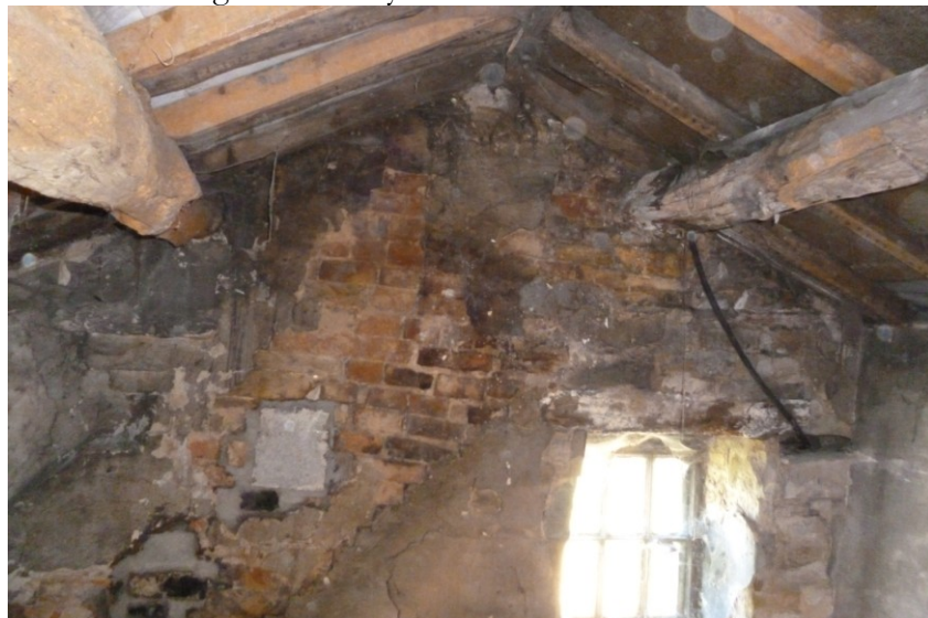
Figure 3 – Riley House internal roof void.
