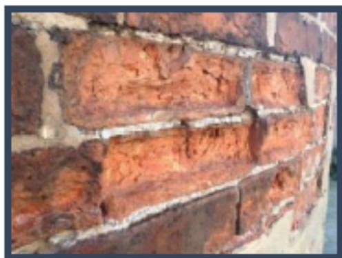
The mortar should be softer than the material it is being used to bond. Using cement, which unlike lime mortar is not soft or porous, will trap moisture in brick or stone which can then cause frost damage and the deterioration of the bonded material.
