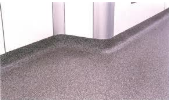
Example of resin floor
