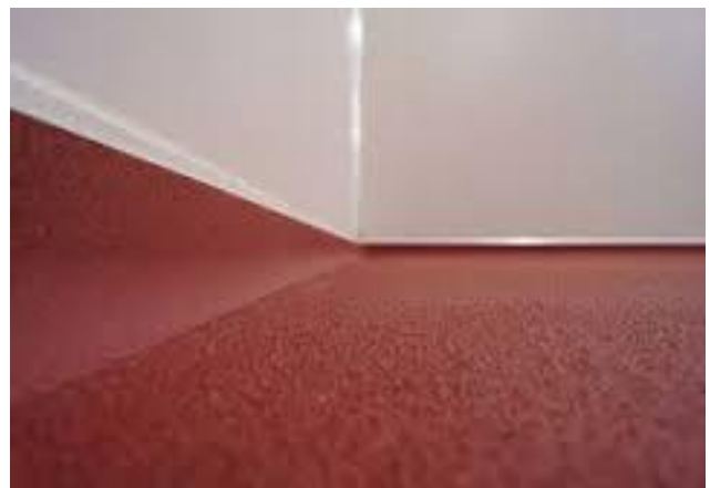
Example of slip resistant floor
