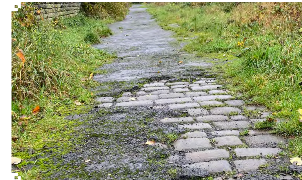
Renew surface of Viaduct in line with heritage and structural advice.
