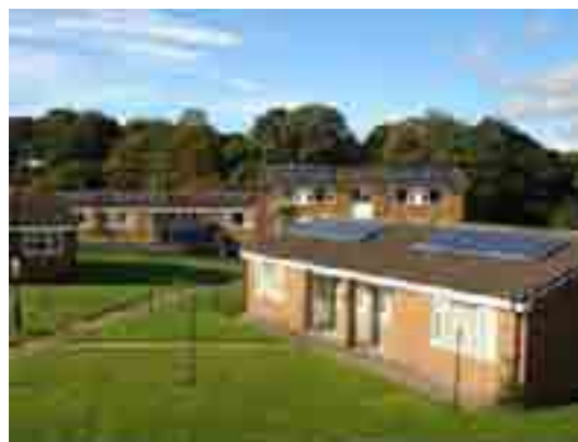
Fernside solar village: 100 solar PV panels
