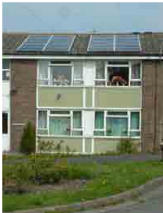
Solar PV panels installed at Primrose Hill
