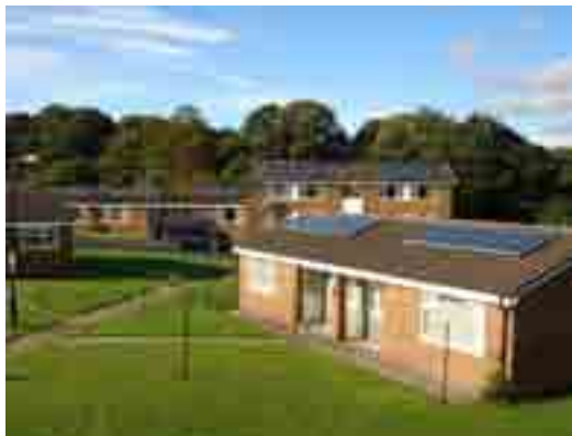
Photo: Sustainable Energy Installations
