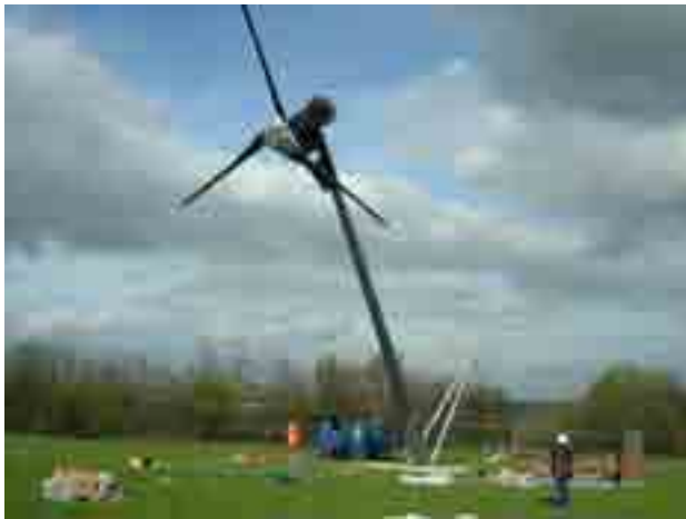
Raising one of the wind turbines
