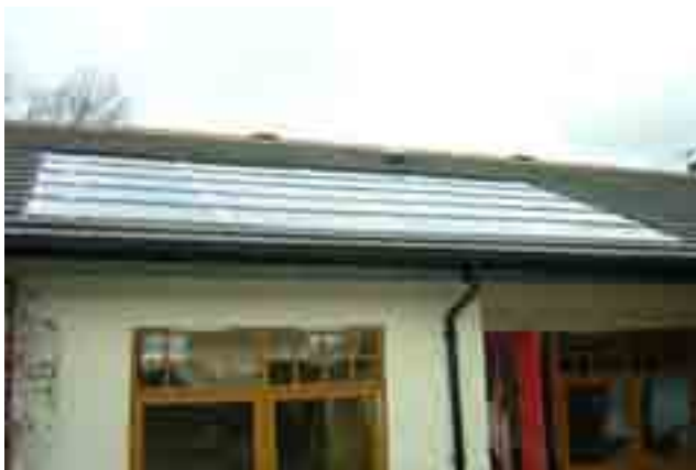
Installation of one 2.5kWp array at Elm Grove sheltered home
