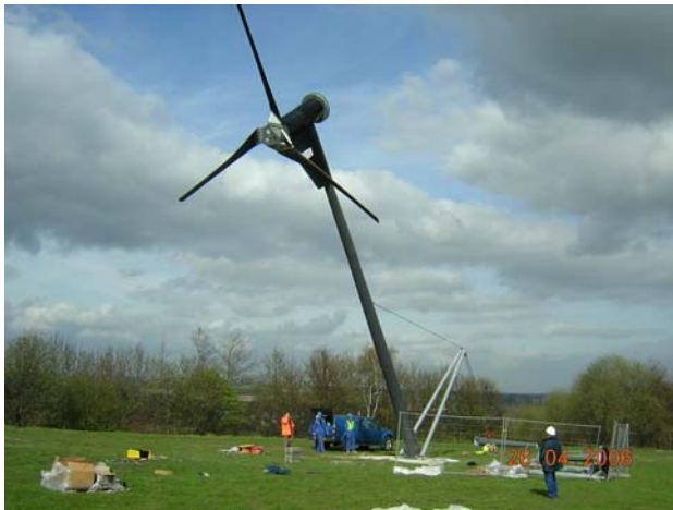
Raising one of the wind turbines
