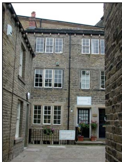
Above: Refurbishment of premises in Wormald's Yard
