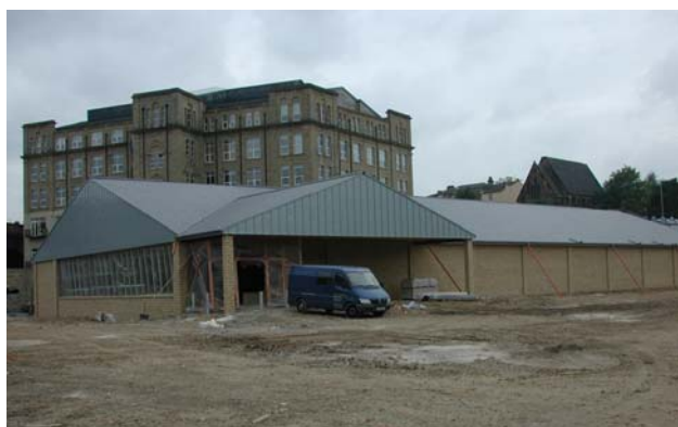
Lidl, Bradford Road, under construction
