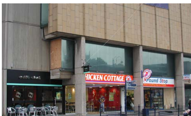
Yorkshire House, South Street
