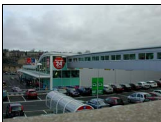
Left: New Tesco Bridge Link
