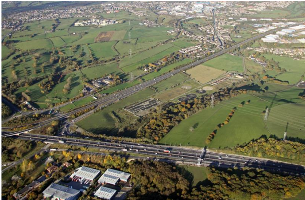
Aerial photograph of the site looking north-west towards Oakenshaw, Euroway and Low Moor
