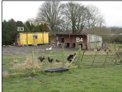
Buildings B3 and B4
