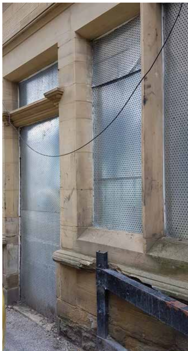
Fig 21. Secondary exit from ground floor lounge area 1 to be blocked up. Steel protection barrier to be removed and damaged stone detail replaced
