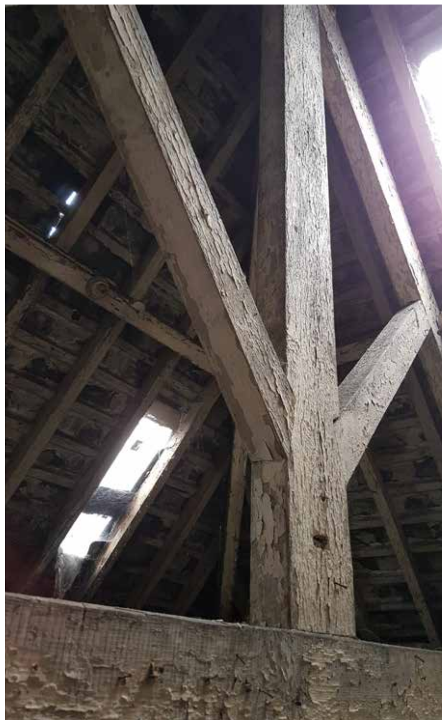
Fig 33. King post roof truss to be modified
