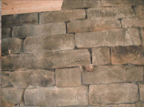
P12 Internal gaps in masonry, barn
