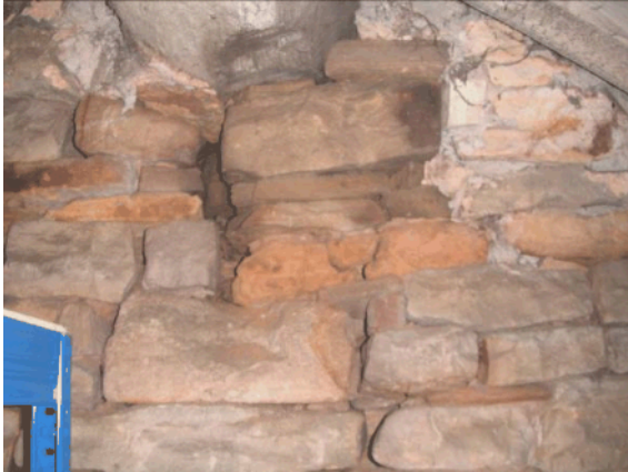
P11 Internal gaps in masonry, barn
