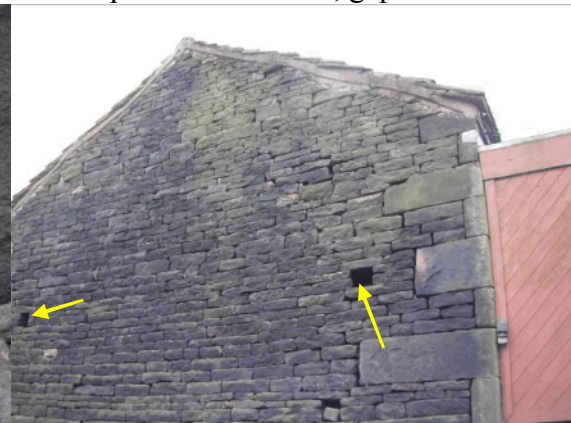
P6 north gable, gaps in masonry
