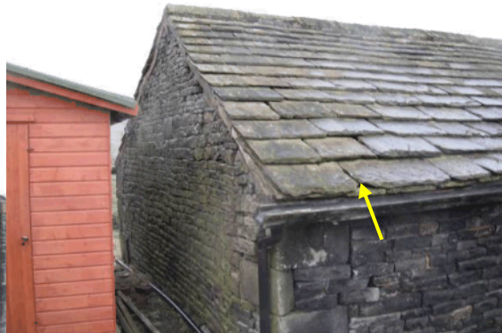
P2 East side and south gable, gaps under tiles
