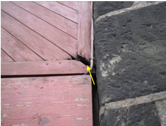
P5 North aspect link section, gap under cladding
