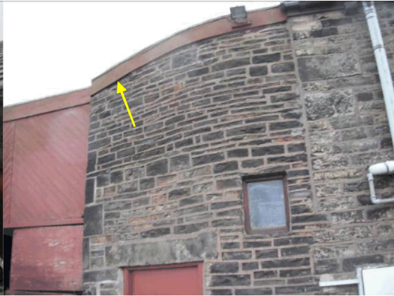
P4 North aspect link sections, gap under fascia
