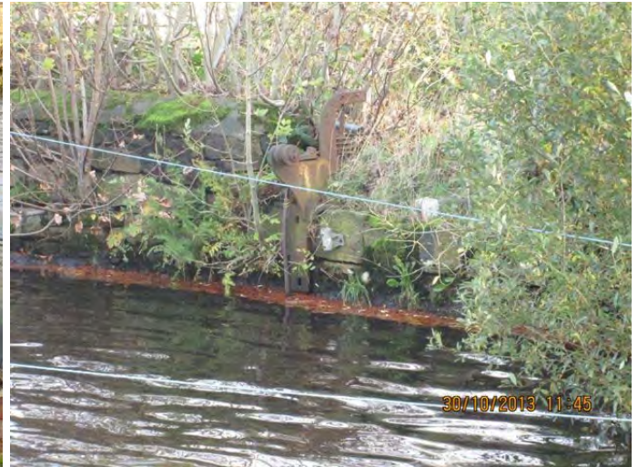
20. Sluice control in intermediate dam.
