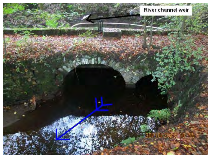
2. Masonry arch inlet culvert
