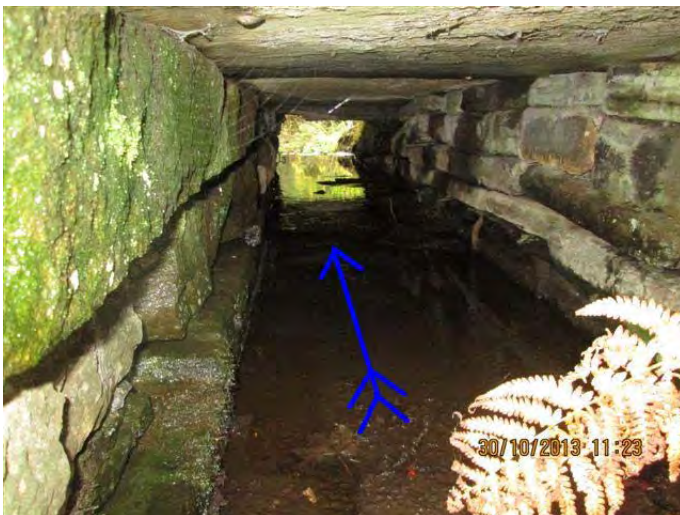
9. Rectangular culvert from overflow
