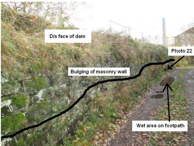
21. Bulging of masonry wall
