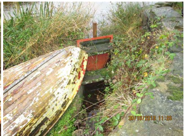
10. Sluice control on left side of overflow
