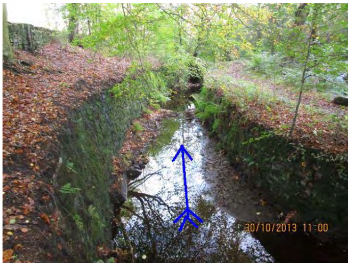
3. Masonry lined inlet channel
