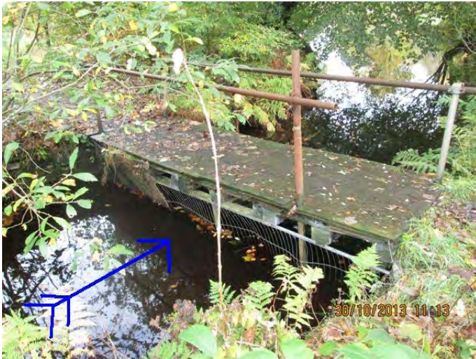
7. Scaffold access bridge over inlet channel
