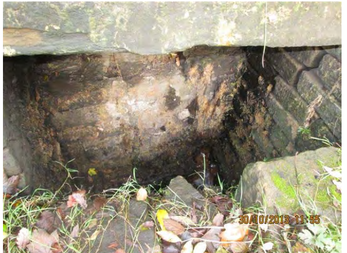
22. Chamber in masonry retaining wall
