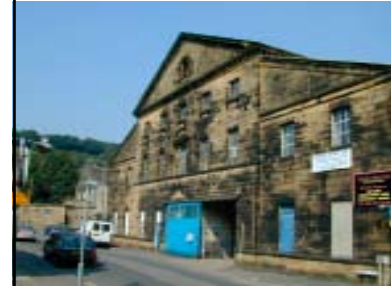
Grade 2* Milnsbridge House viewed from Dowker Street
