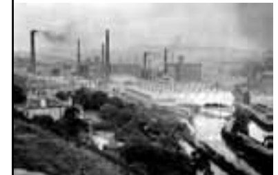
Early photograph of Milnsbridge showing the industrial landscape and the many mill chimneys
