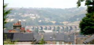
The grade 2 listed viaduct which carries the railway across the valley
