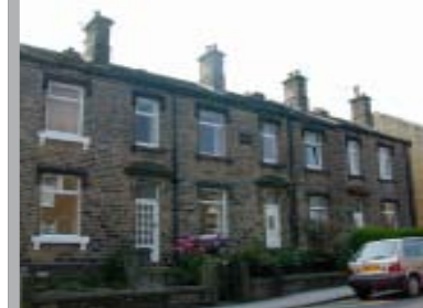
An attractive terrace of late 19th century houses
